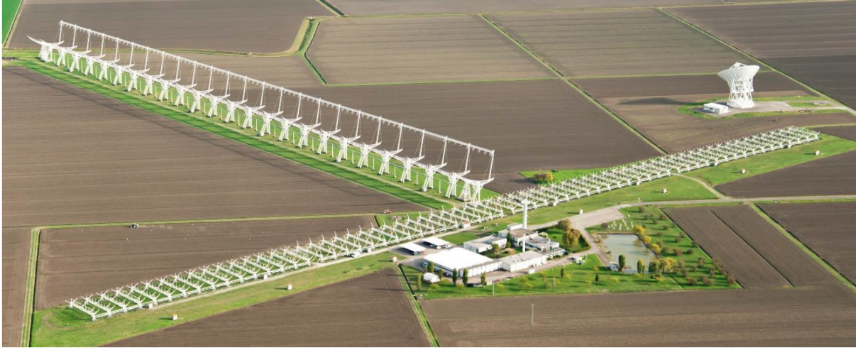
Figure 1: Top view of the Northern Cross radio telescope with the two perpendicular arms along the East-West and North-South direction.
