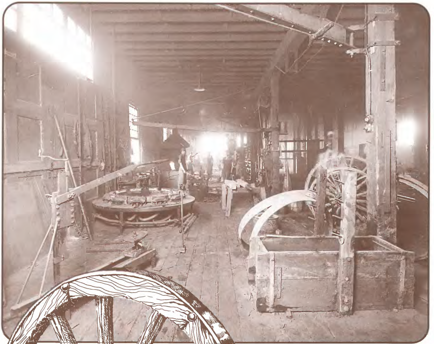
Interior view of a blacksmith shop where steel tires are being made for wagon wheels. Sometime between 1890 and 1910. Photographer unknown. (X-24574)
